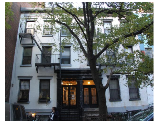
285 and 287 East Third Street
