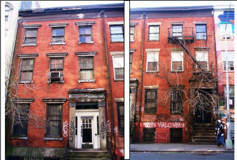
326, right, and 328 East Fourth Street, prior to alteration
