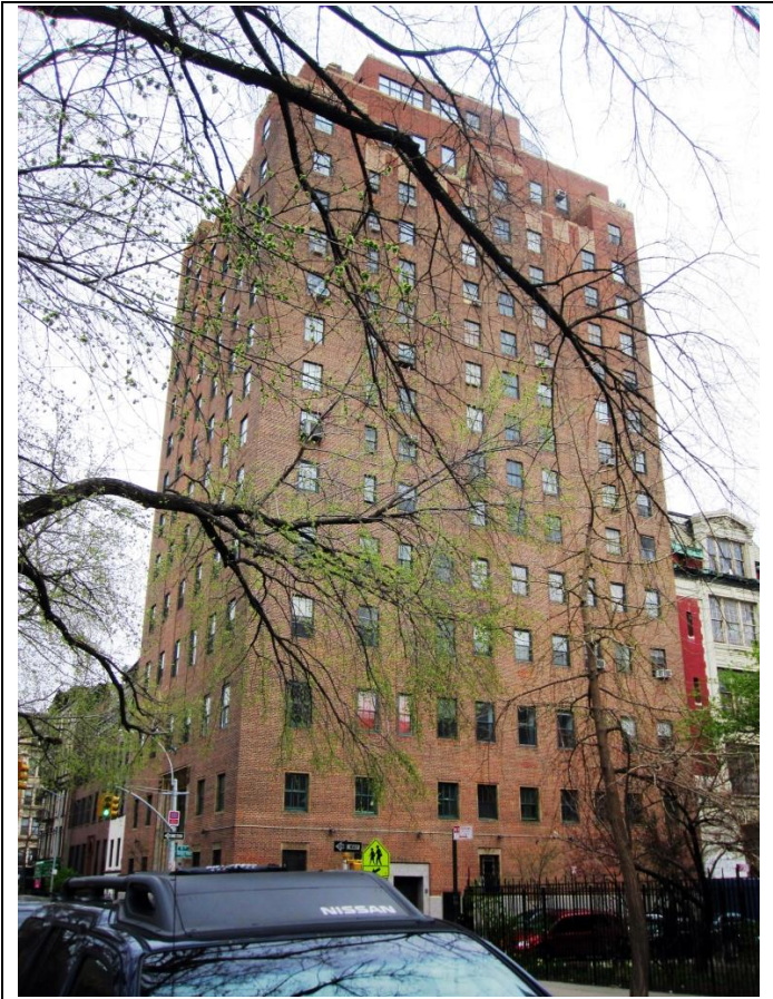
Christodora House, south elevation
